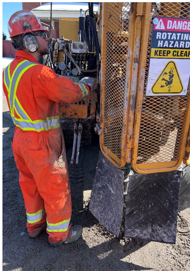
Photo #6- Augering out silty clay in BH-04
